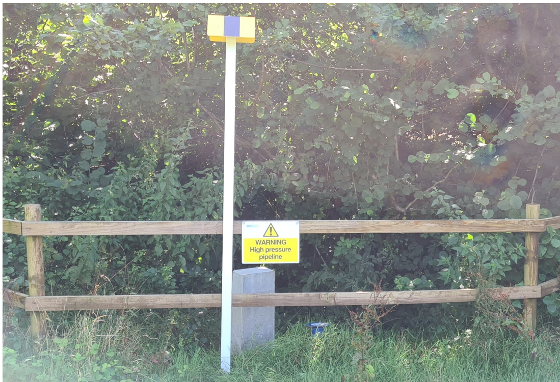
Figure 4: Examples of fencing off affected areas and additional pipeline marking
