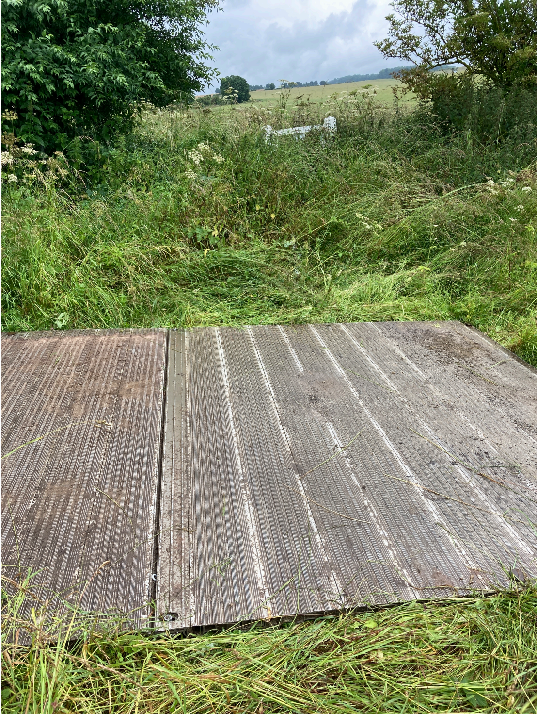
Figure 3: Aluminium protection plates installed above ground as temporary protection
