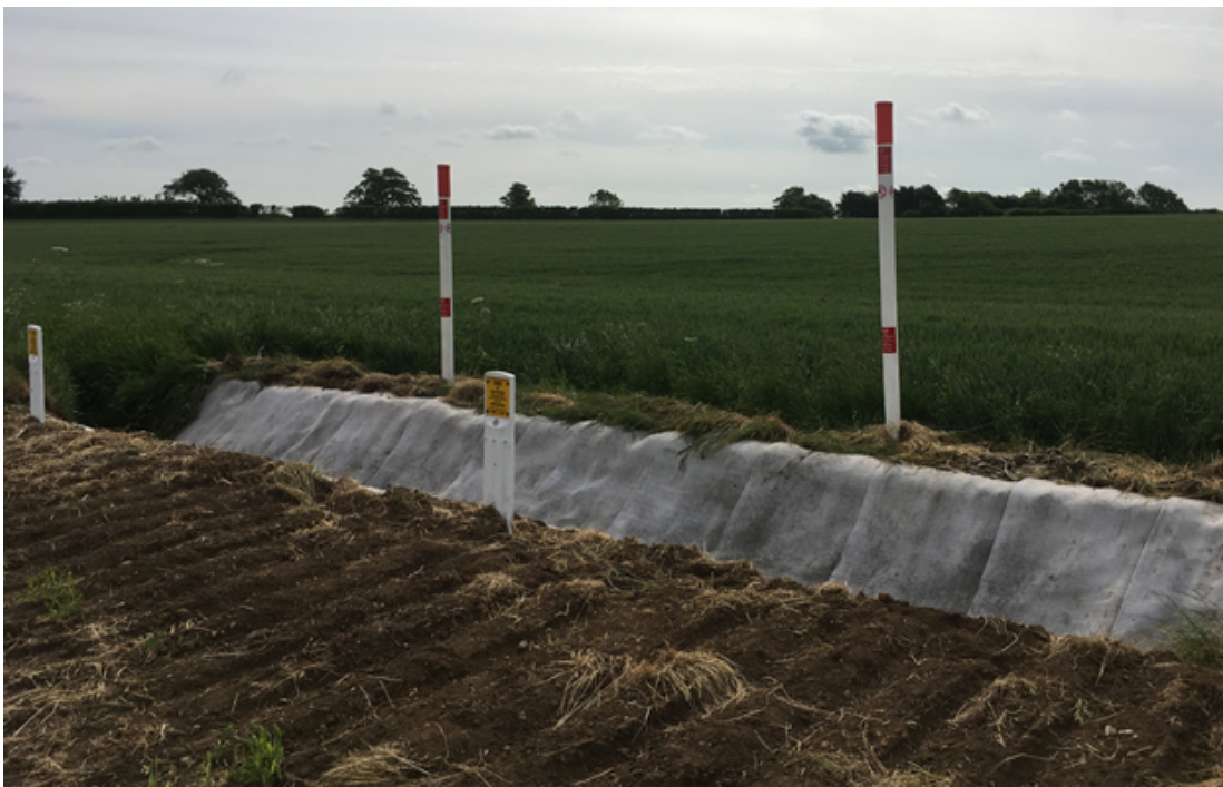
Figure 7: Ditch remedial using concrete canvas and additional marker posts
