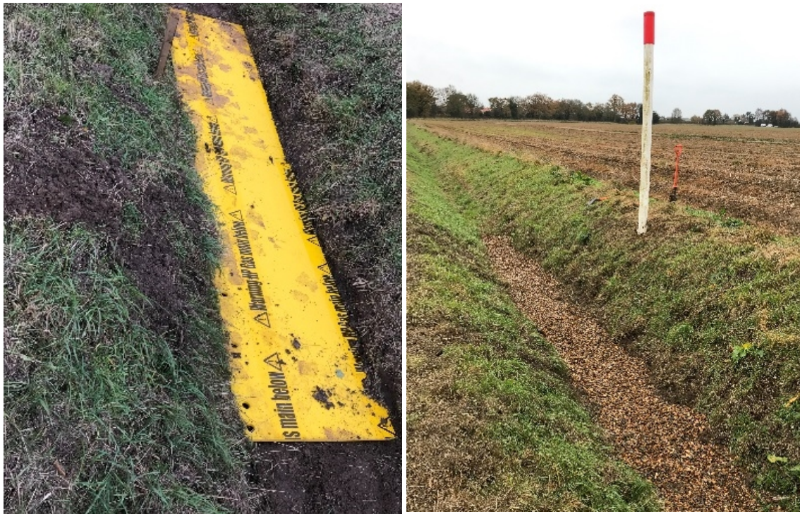
Figure 1: Left - Plastic ditch board installed over pipeline with reduced depth of cover Right - Depth of cover reinstated, note the marker post at the ditch crossing
