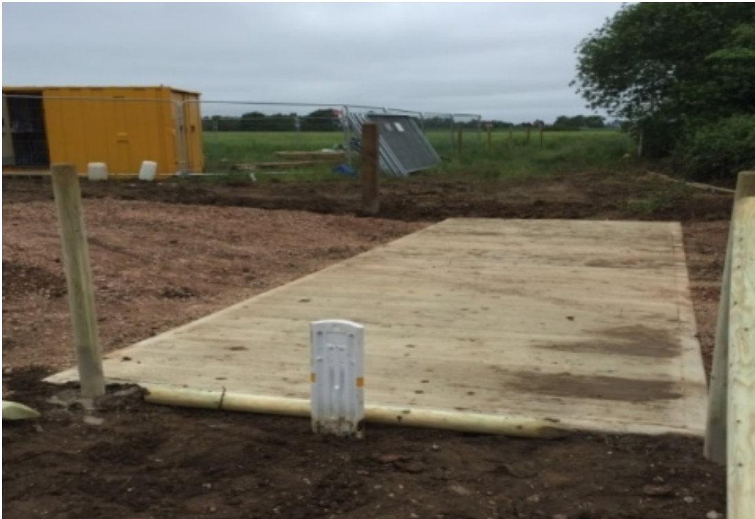
Figure 6: Protection slab and additional markers posts
