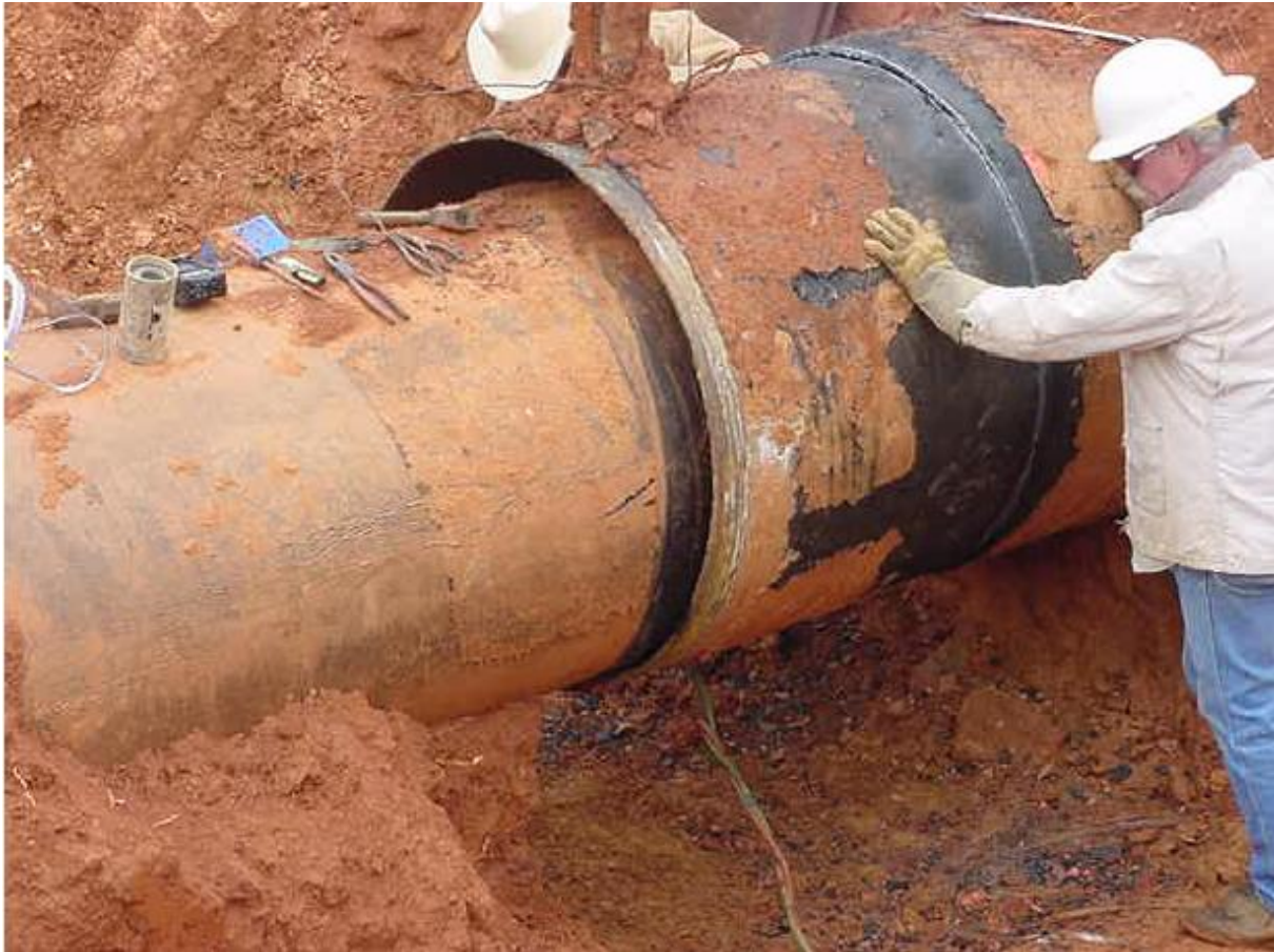
Figure 5: Pipeline and sleeve (NACE)
