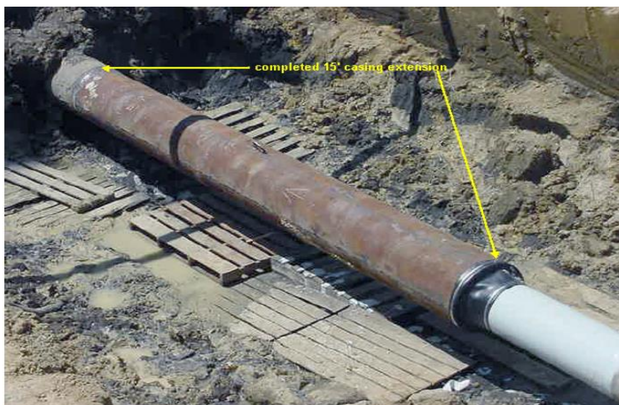
Figure 7: Sleeve extension completed (NACE)
