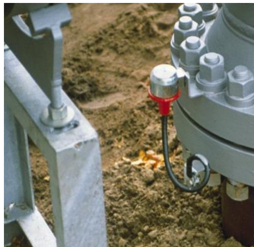
Figure C2 Zone 2 only certified spark gap device
