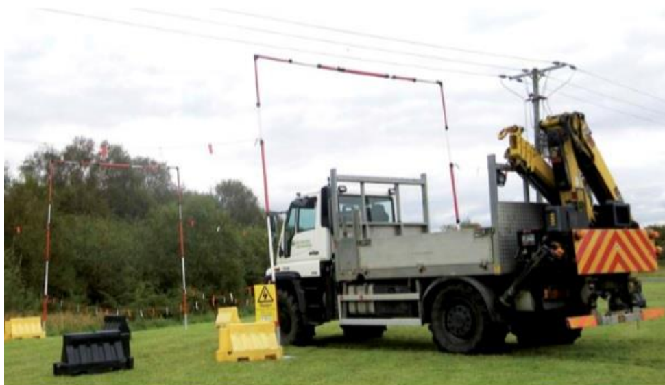
Figure 7 Typical construction arrangement at overhead powerline crossing taken from GS 6
