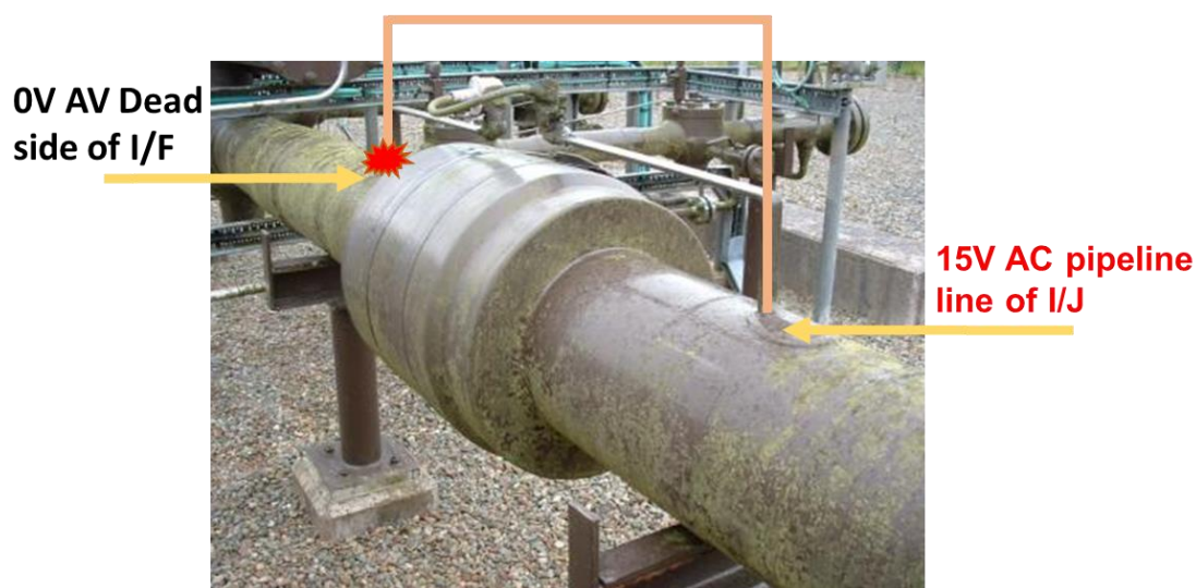
Figure 13 Spark risk on short circuit of I/J with a.c. voltage present
