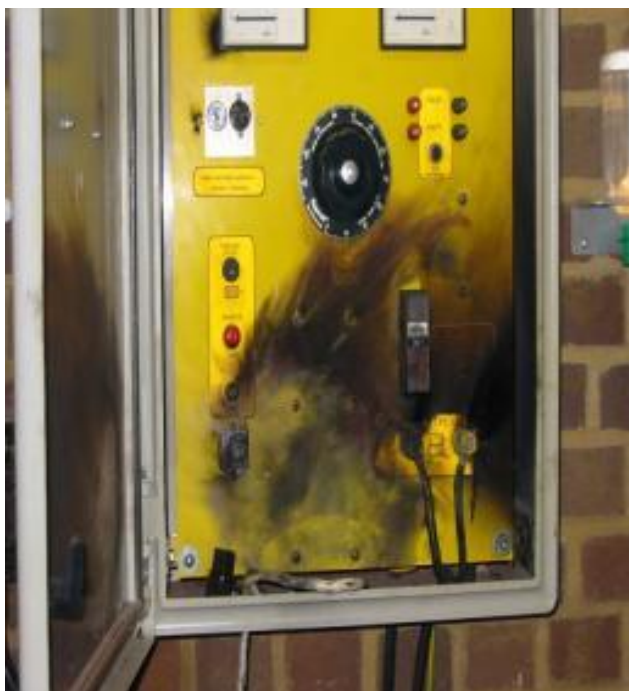
Figure 17 Damage to CP T/R unit as a result of arc strike on pipeline
