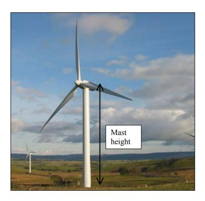
Based on the study, the appropriate exclusion zone (distance from base of the wind turbine mast to the edge of the pipeline) has been identified as 1.5 times the turbine mast height.
