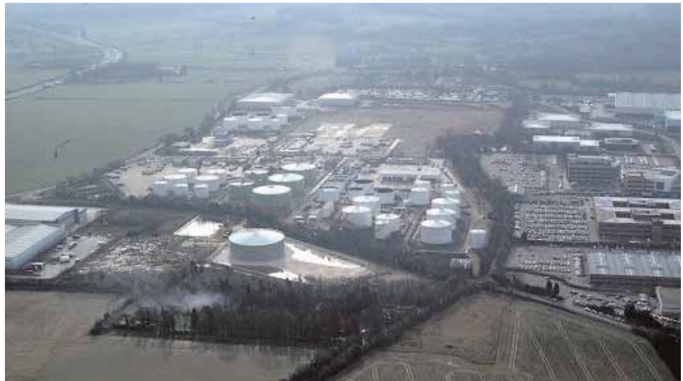
Figure 7 The area prior to incident
