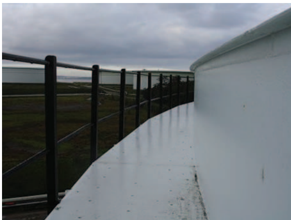
Figure 3. Top grider (walkway) in floating roof tank
