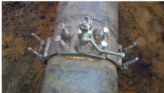
Figure 4.3: Circumferential clamp with pre-welded valve
