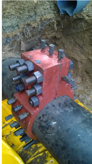
Figure 8.5: Epoxy filled split tee
