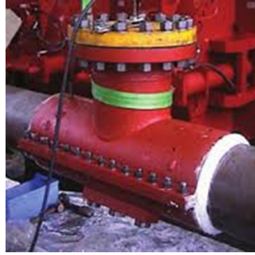
Figure 8.2: Grouted tee
