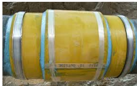
Figure 8.4: Composite wrap
