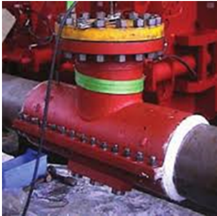
Grouted tee (by DNV)
