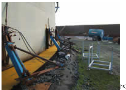
A 54m storage tank slipped sideways on its jacks
