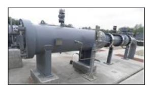
The original GFSA design incorporated a secondary latch design. Under trial conditions, it was found to be possible to open the filter door with residual pressure inside the vessel. The door was designed to release the door holding elements inside the door with a 10 degree movement of the door operating lever; a further 5 degree movement disengaged the secondary latch fingers visible on the door from the blocks on the filter body.
