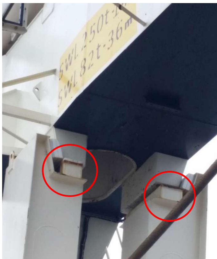
Location of Teflon pads on crane rest.
