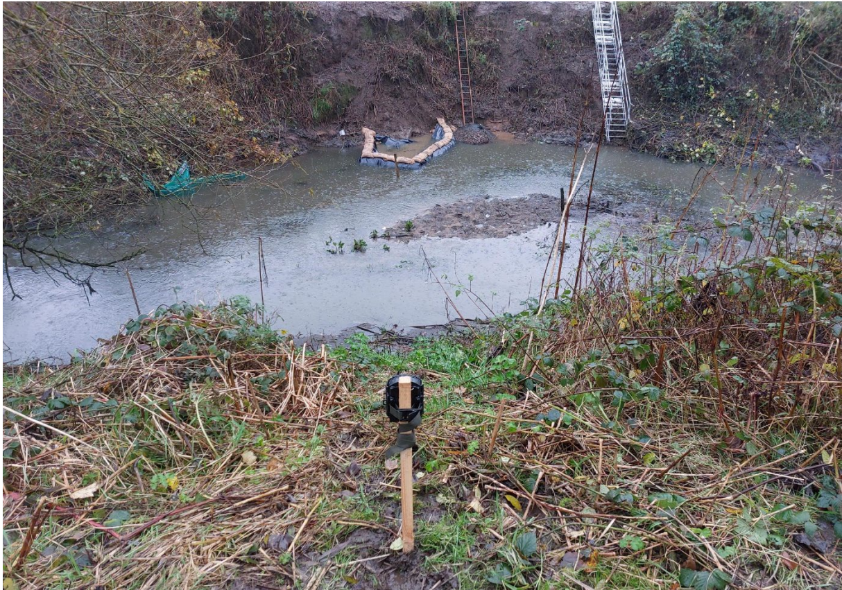
Figure A-10: Temporary Cofferd Dam Installation
