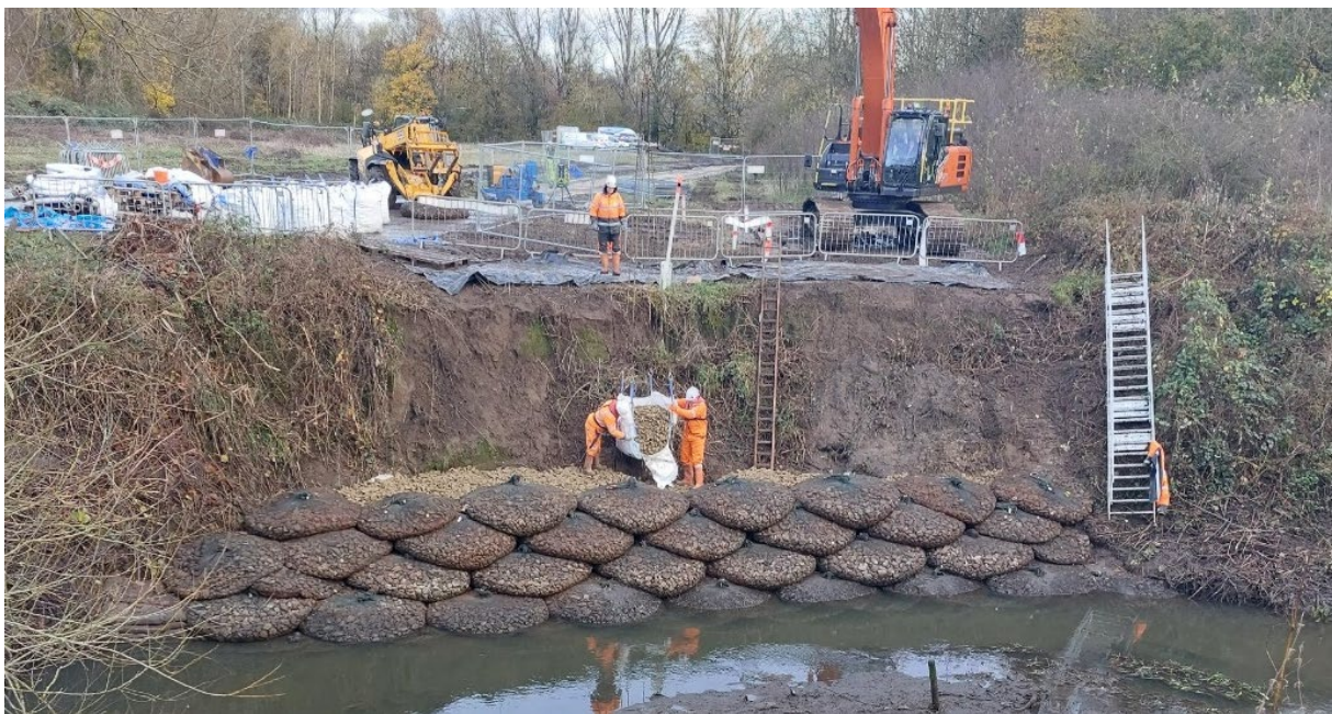
Figure A-11: In Progress Bank Reinforcement with Rock Bags and Backfill
