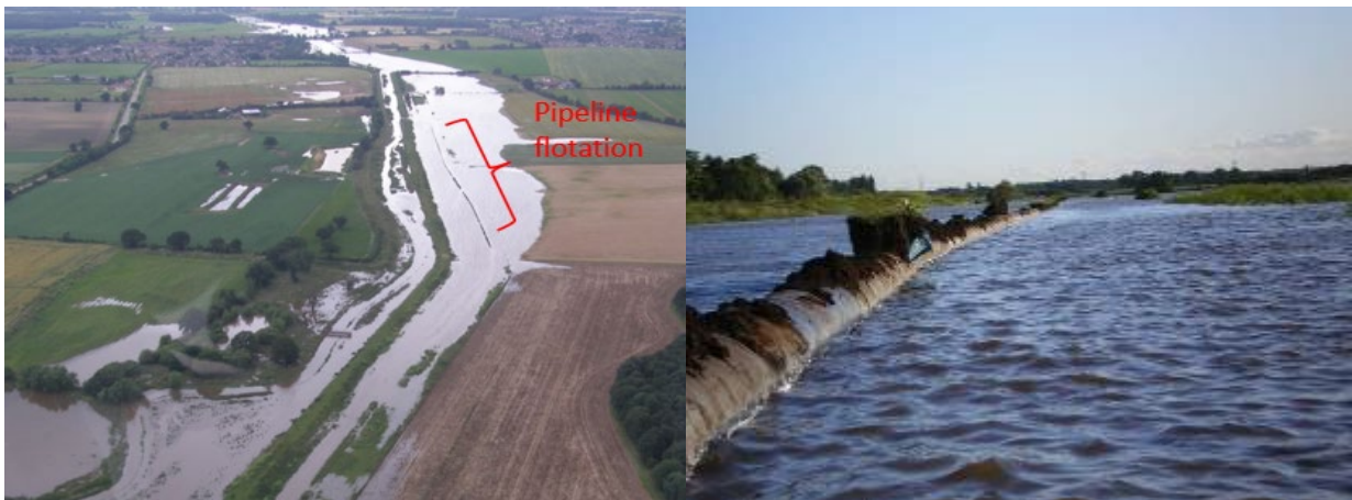
Figure A-13: Pipeline Buoyancy
